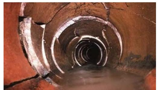
Figure 1 - Cracked and leaking sewer pipe
