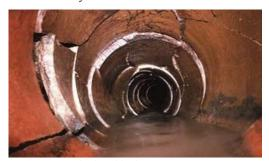
Figure 1 - Cracked and leaking sewer pipe
